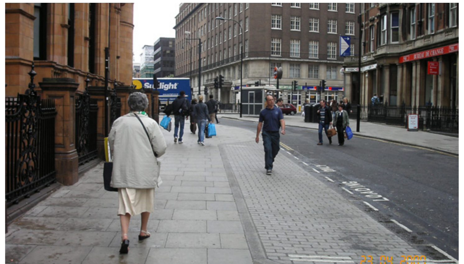
Image 4.11: Street after addition of level loading pads
