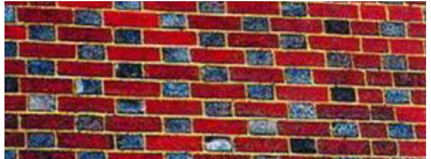
Image 7.2: Flemish bond handmade red brickwork with burnt headers (image from RBBC Character and Distinctiveness SPD)
