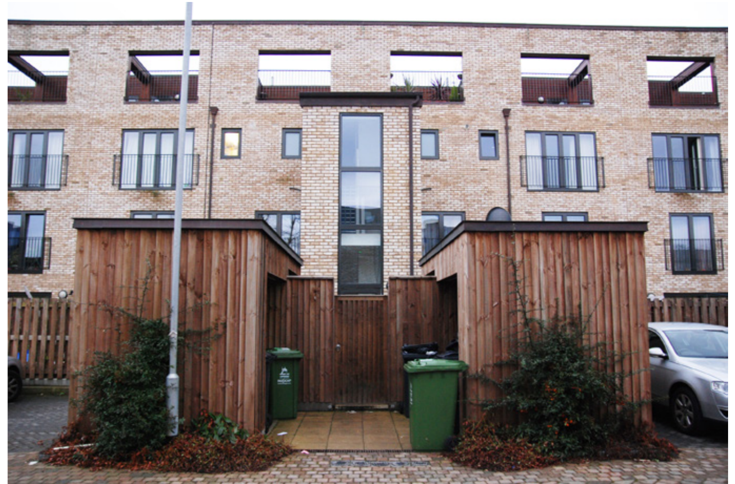
Image 6.6: Servicing is well-integrated into the design of the development within the rear parking court
