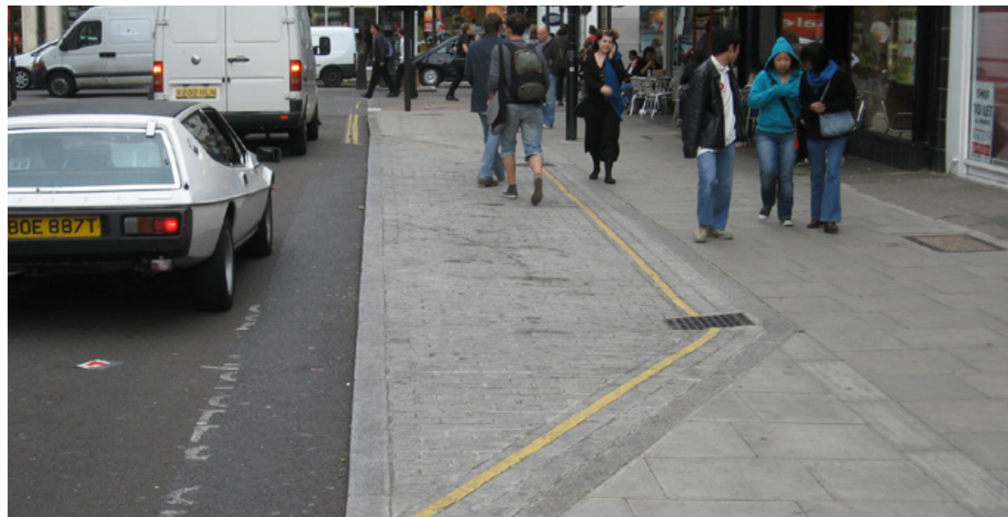
Image 4.9: Level loading pads
