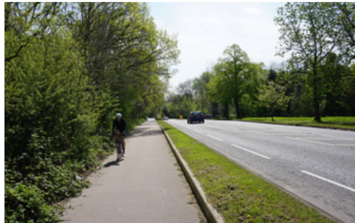
Image 1.8: In some places a bi-directional shared walking/cycle route already exists alongside the A23
