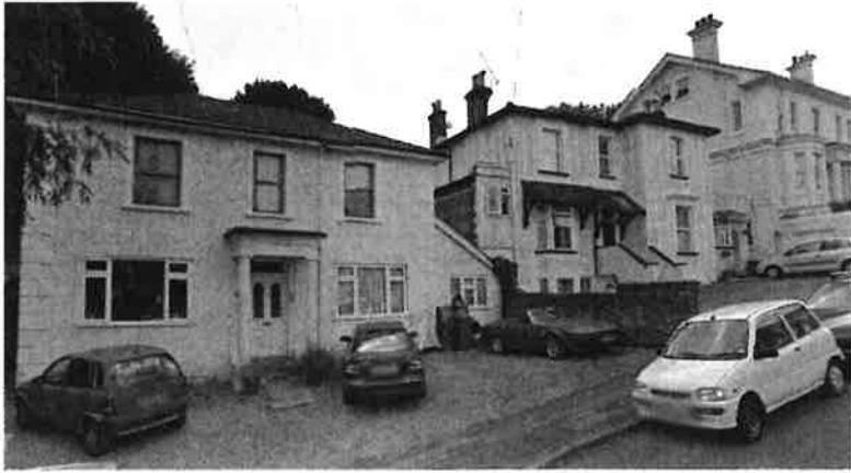
Loss of landscaping and inappropriate alteration can be an issue.
