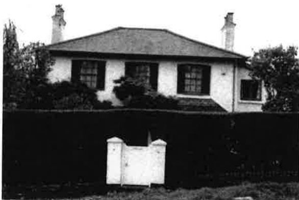
No 10 is early 19 th century grade II listed building
