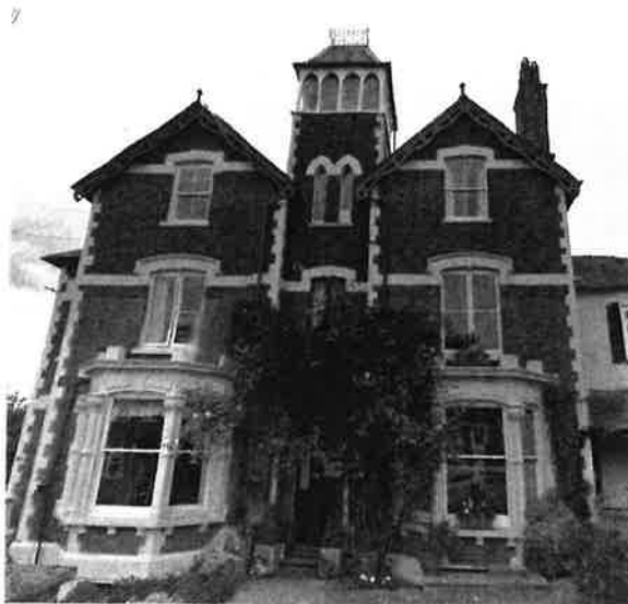
Ridgeway Road is characterised by Victorian gothic brick houses.
