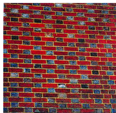
Flemish Bond Handmade Red Brickwork with Burnt Headers
