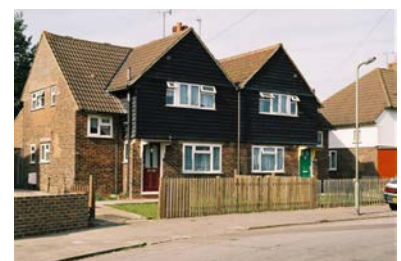
Brook Road, Merstham - example of weatherboarding, painted a dark colour, which does not reflect local styles
