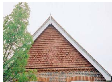
Handmade tile hanging used at a recent development in Reigate
