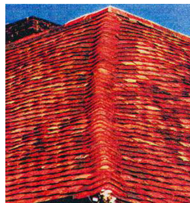
Handmade sandfaced plain clay tiles with half round ridge tiles and bonnet tiles to hips
