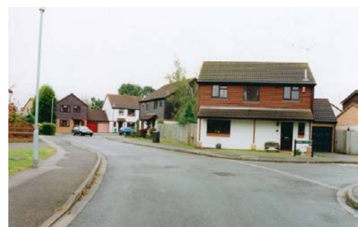
Parkhurst Road - Horley painted timber boarding does not reflect materials used historically.
