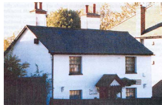
Example of Victorian Stucco
