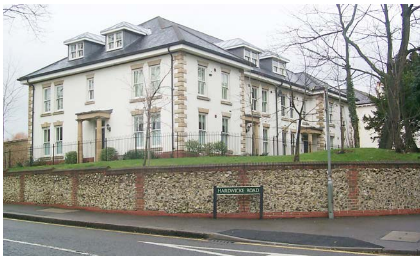
Flint wall at Hardwicke Road/London Road, Reigate
