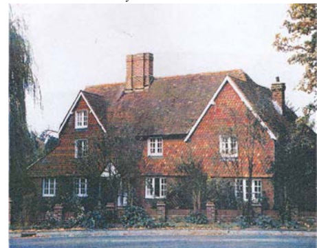
Typical Asymmetrical Wealden vernacular Farmhouse 50 degree pitch clay tiles and decorative tile hanging
