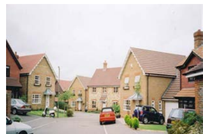
Osier Way, Banstead - Material Palette is too varied and the layout is too cramped
